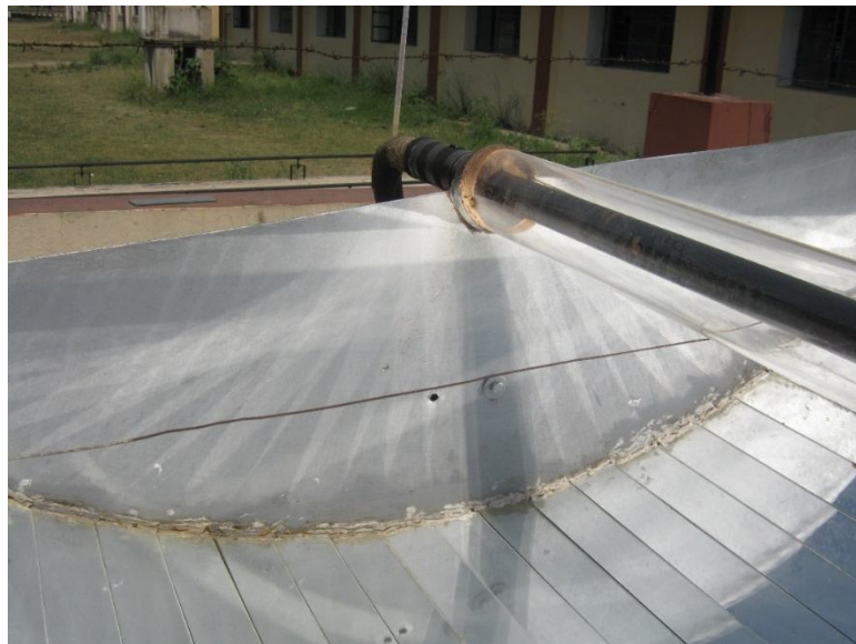
Figure 4.2: Reflection of solar radiations to Receiver tube via Reflector
