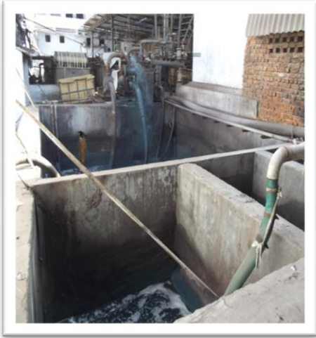
Collection cum Equalization Tank
