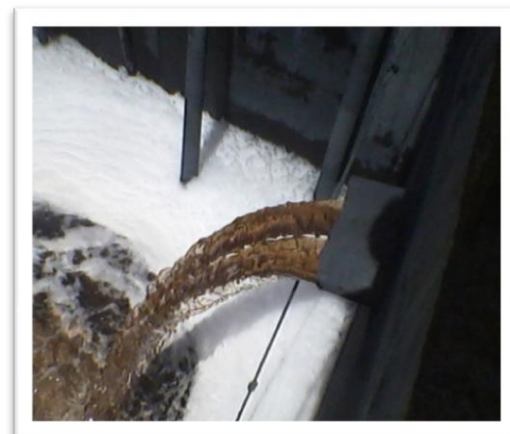
Final Treated Effluent sump
