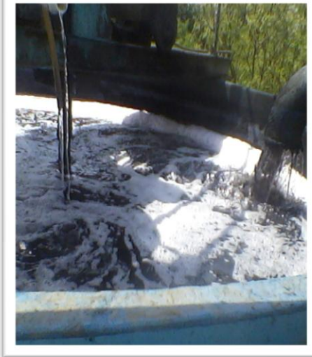
Inlet to flocculator Mixer
