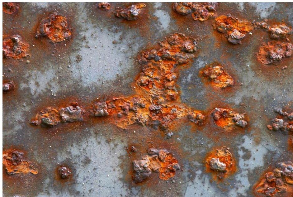
Figure 1.9 Intergranular Corrosion (Source: steelfabservices)
