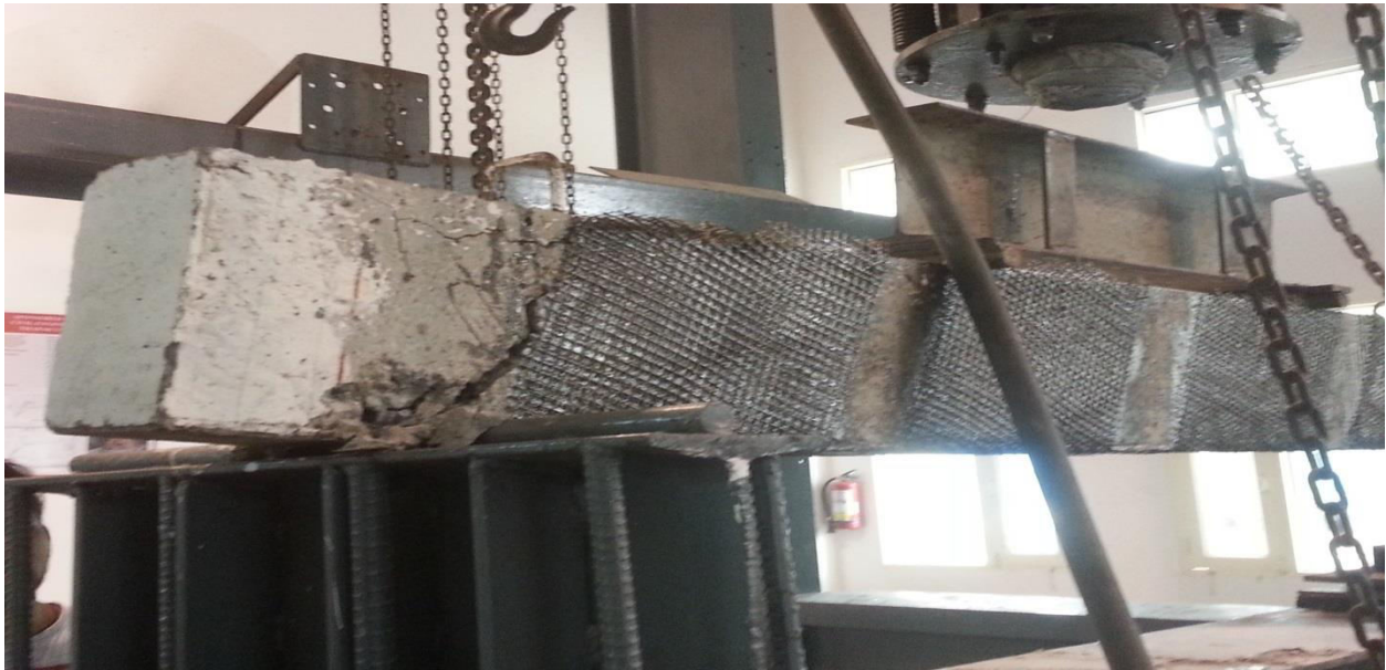
Figure 4.9 Failure and Crack Pattern of Beam Strengthened with no Inclined Strips on Face A
