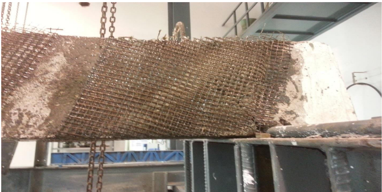
Figure 4.10 Failure Pattern of Beam Strengthen with Inclined Strips on support on Face B
