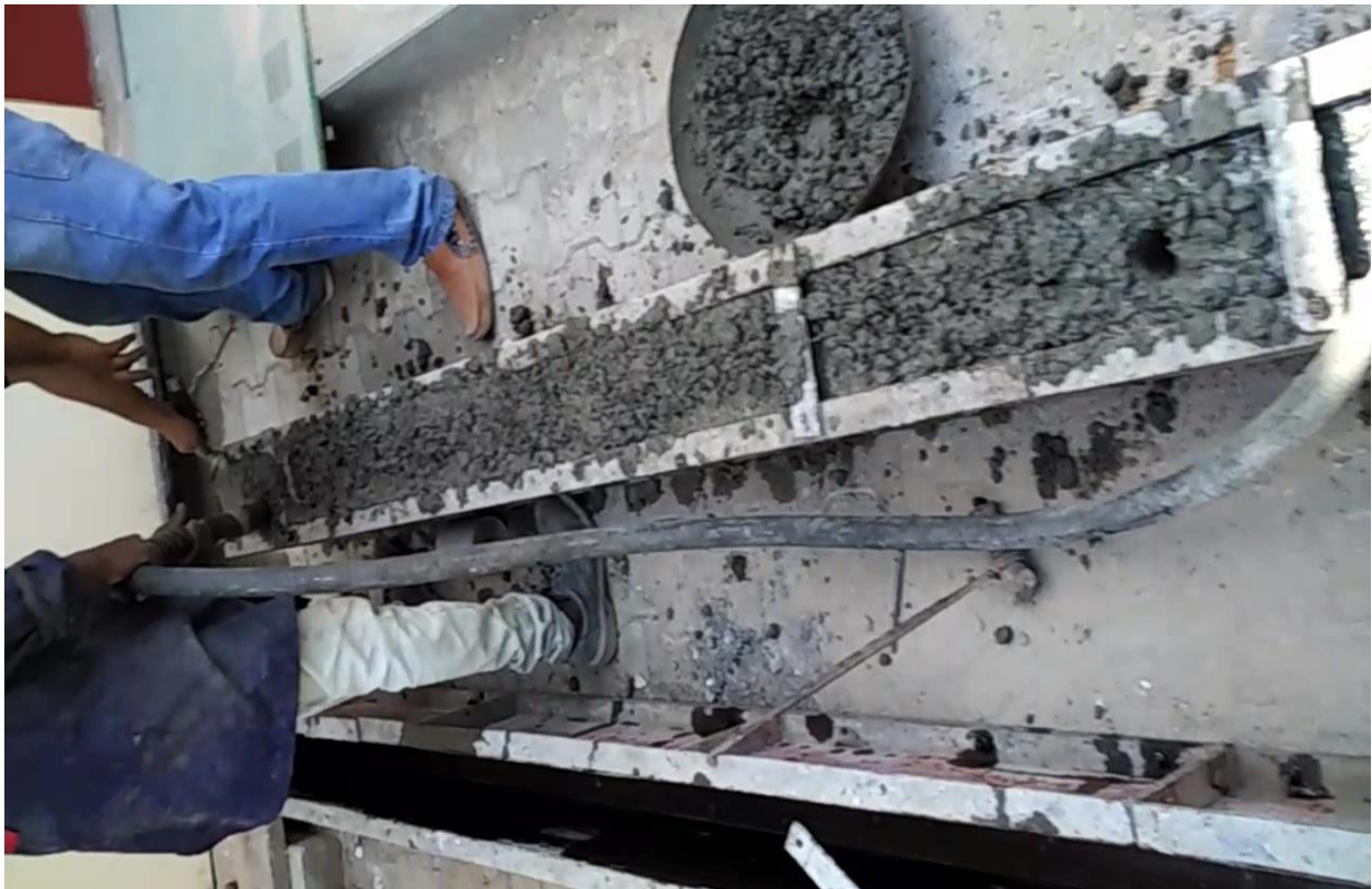
Figure 3.3 Casting of RC Beams
