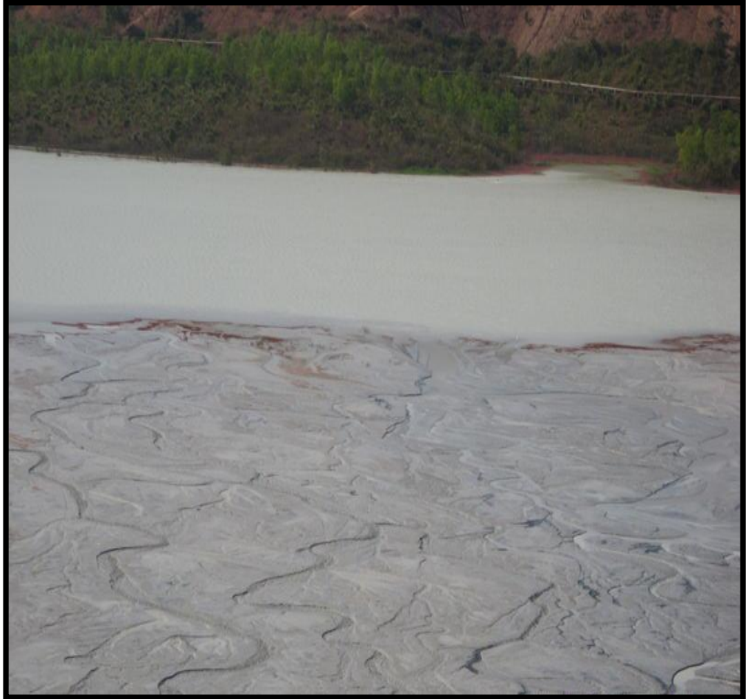
Fig 2.2: Disposal of fly ash in the form of wet slurry to nearby artificial impoundments at NALCO, Damanjodi, Orissa, India.
