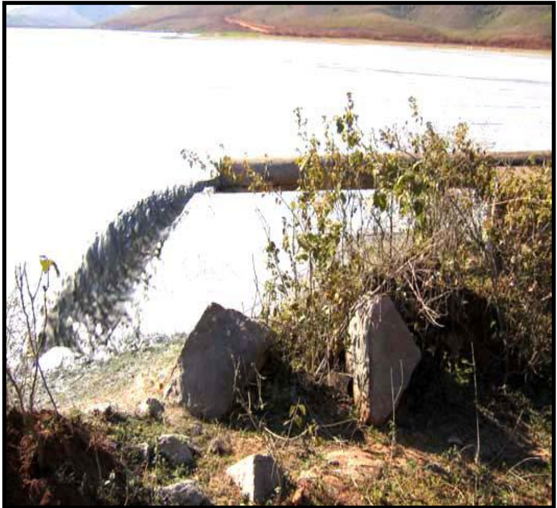
Fig 1.4: Disposal of fly ash in the form of wet slurry to nearby artificial impoundment at NALCO, Damanjodi, Orissa, India.
