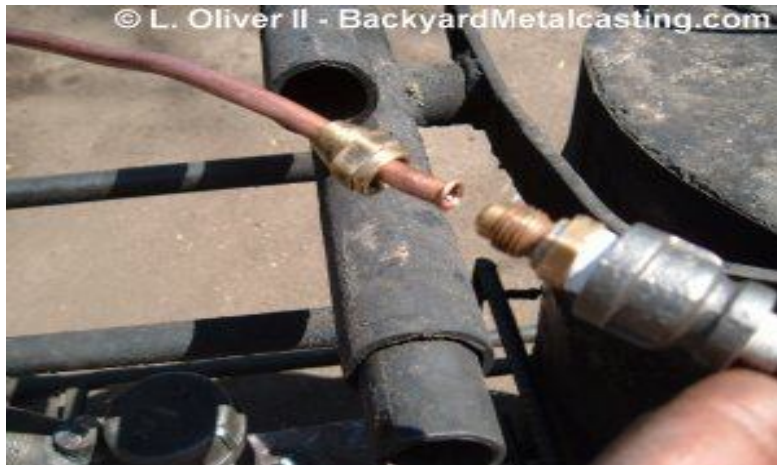
Fig.5.23: Flared connections
