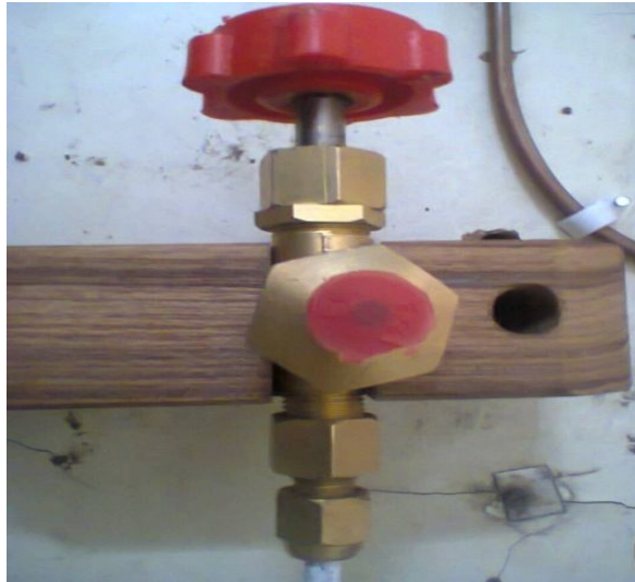
Fig.5.5: Hand operated expansion valve
