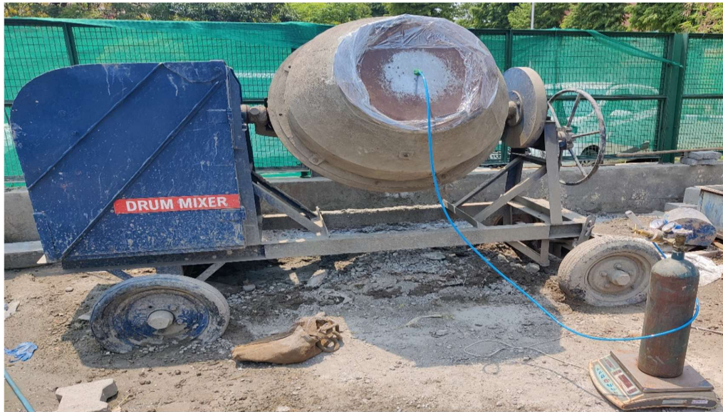
Figure 3. 4 Concrete mixing setup
