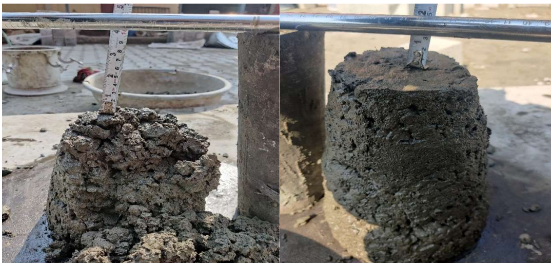
Figure 3. 7 Slump measurement of the concrete
