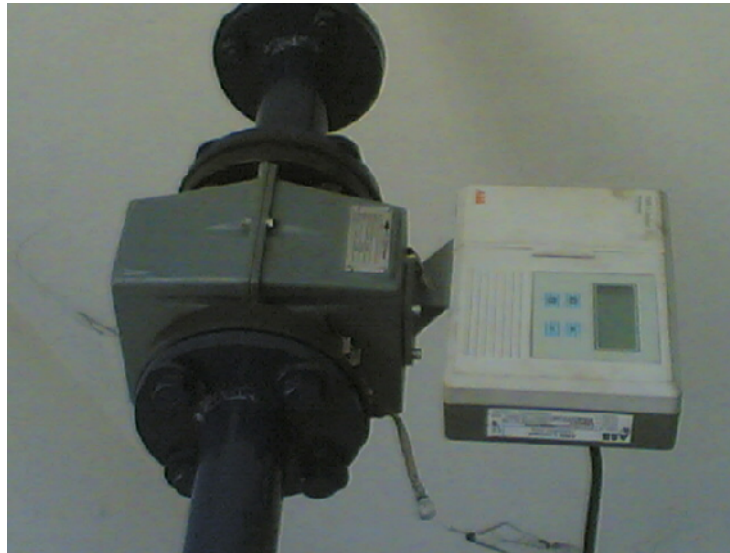
Figure 3.7 Magnetic flow meter
