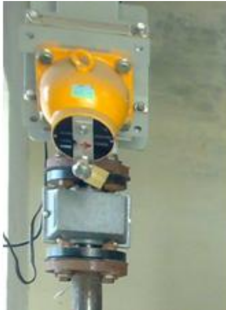
Figure 3.8 Density Monitoring Instrument
