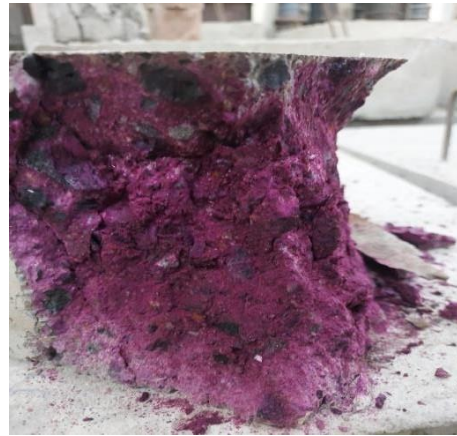
Figure 4.36 Carbonation of mix E75
