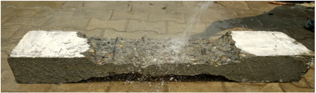
Fig 3.9 (b) Cleaning of beam with water under pressure
