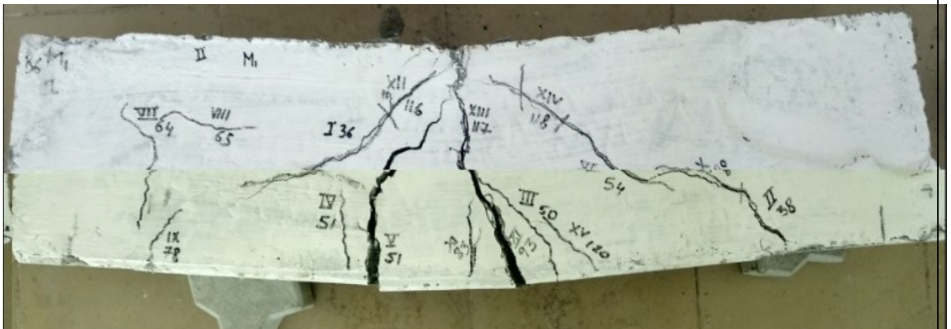
Fig 4.11 Cracking pattern of beam repaired with M1
