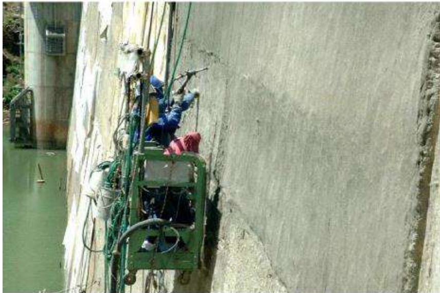
Fig 1.2 Retrofitting of Mitaka Dam by spraying ECC layer (Kunieda and Rokugo, 2006)
