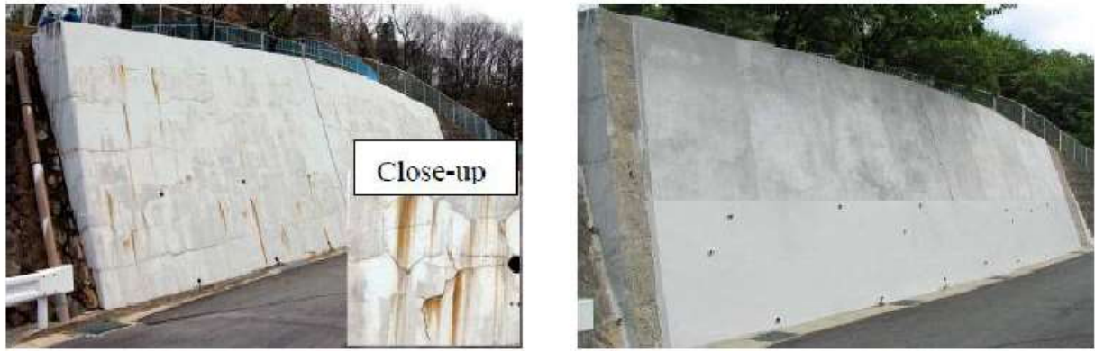
Fig 1.3 Concrete retaining wall before (left) and after (right) (Rokugo et al., 2005)
