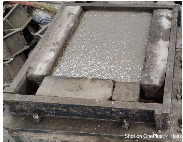
Figure 3.26 Finished and levelled slab
