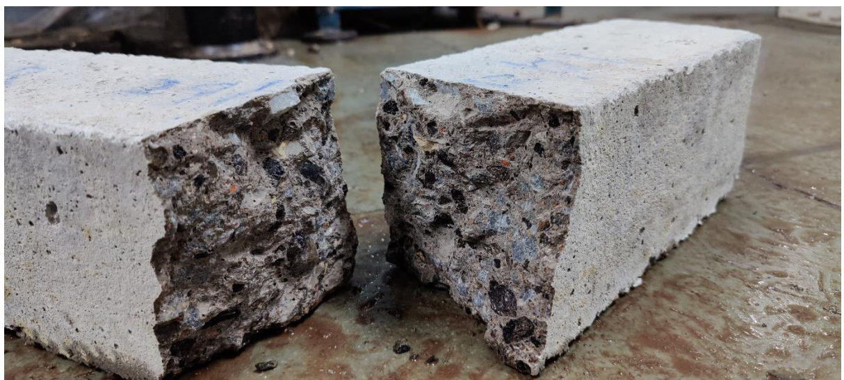
Figure 4.14 Front view of crack pattern in beam specimen used in present study
