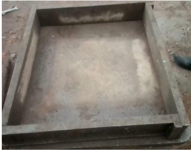
Figure 3.21 Prepared mould of slab
