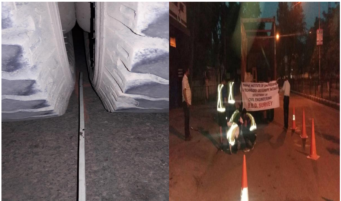
Figure 4.3: Placement of Benkelman Beam apparatus for measuring deflection
