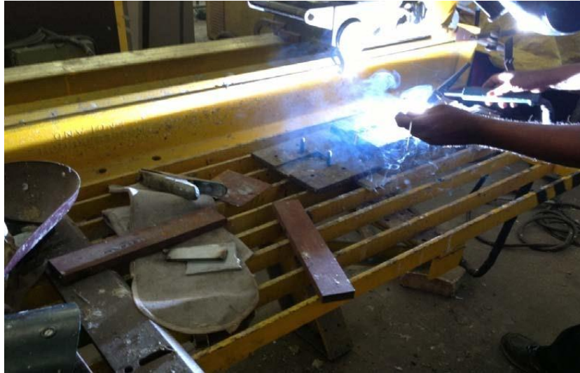
Fig.5.14 Welding in progress
