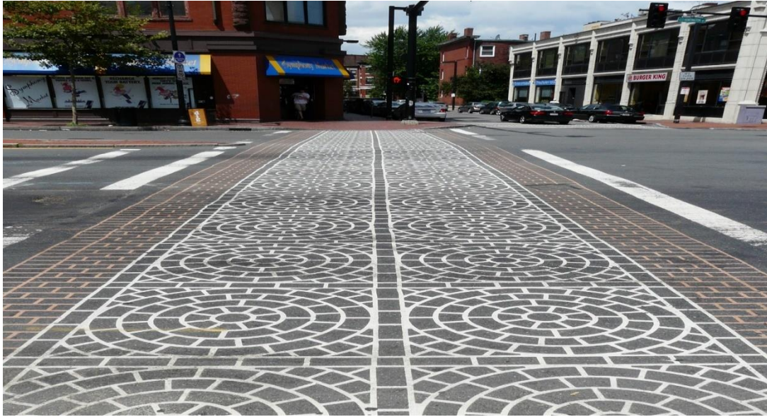
Figure 9.6 Showing Texture of Crosswalk Surface
