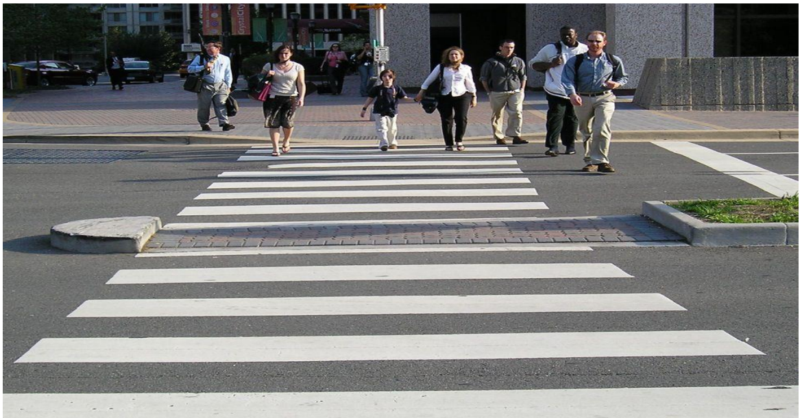
Figure 9.5 Showing Ideal Crosswalk Marking Condition
