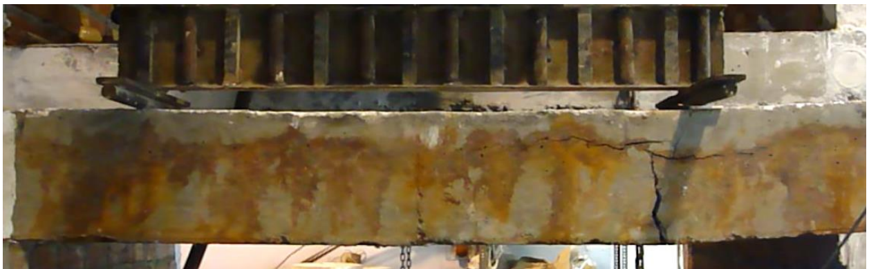
Figure 4.21 C-40 Beam showing large vertical crack
