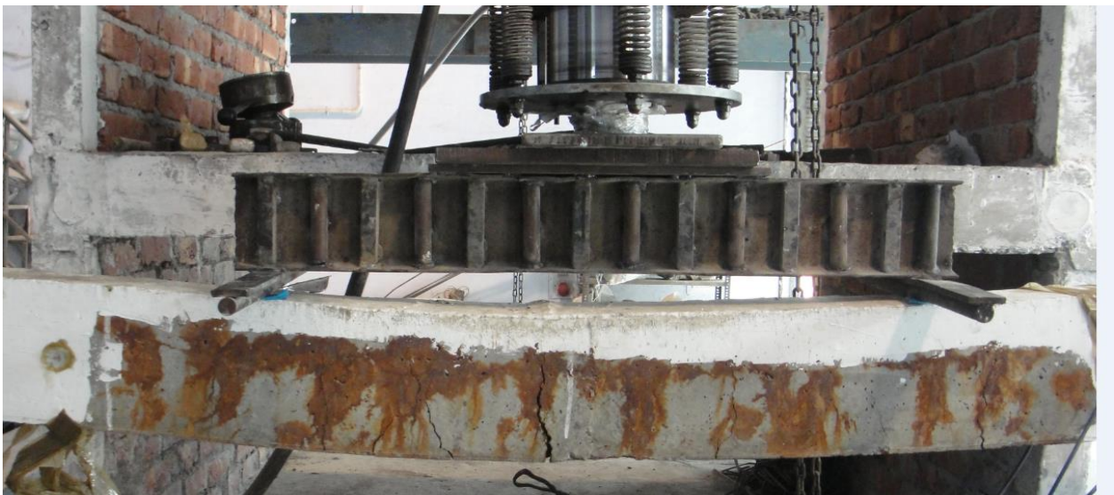
Figure 4.19 C-30 Beam showing large vertical crack near the centre of beam
