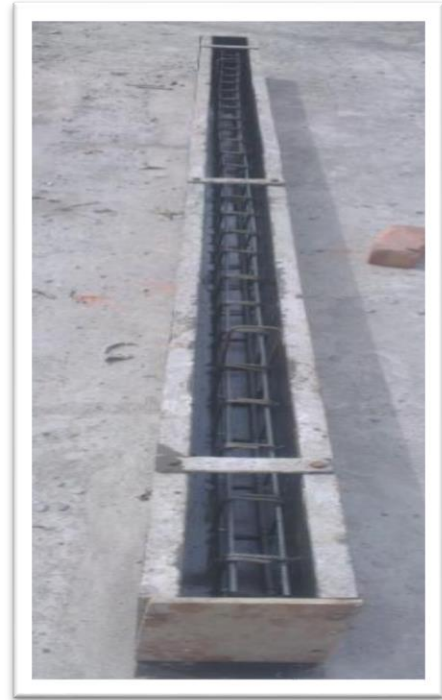
Figure 3.6 Beam mould with reinforcement cage
