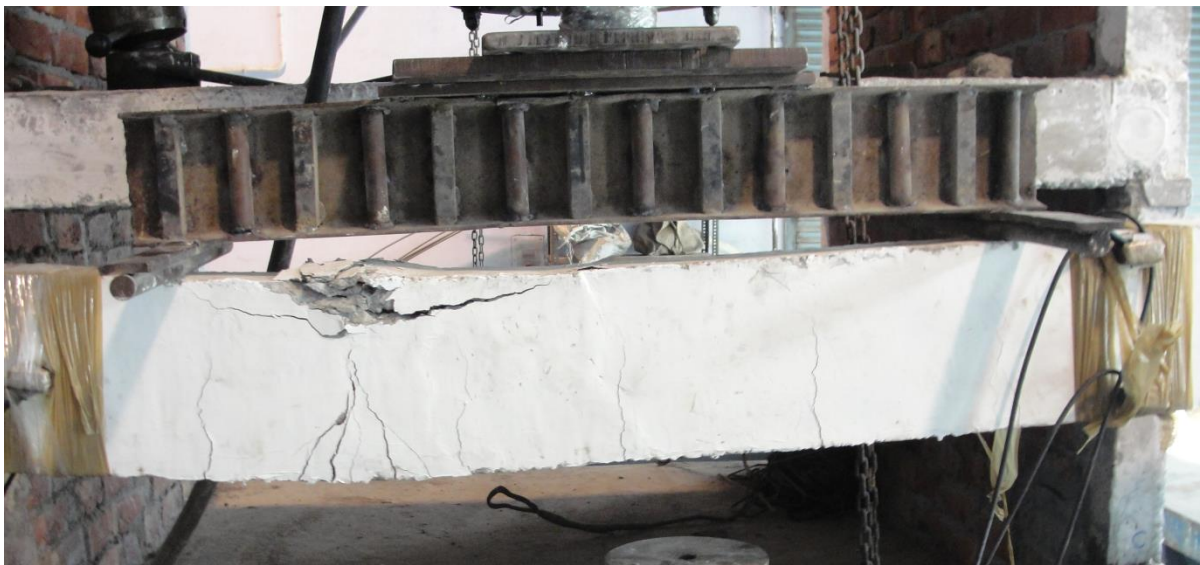
Fig 4.15 Flexure Cracks on side face of C-0 beam
