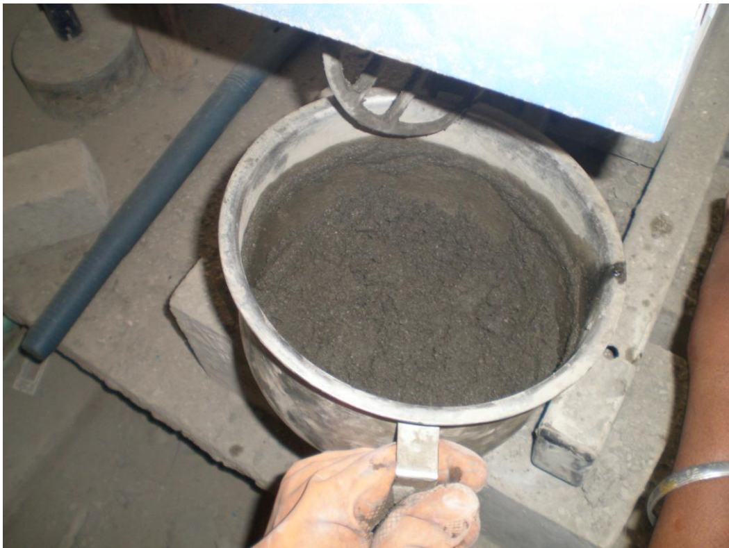
Figure 3.5: (b) Mixing of material for mortar cubes in mixture machine
