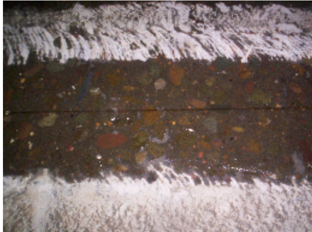
Fig 4.2 Beam surface after grinding & priming
