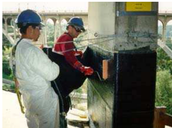
Fig 1.2 photo showing process of column wrapping
