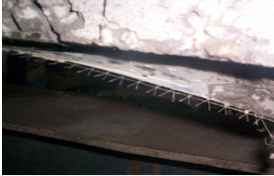
Fig 4.16 Photo showing debonding of sheet
